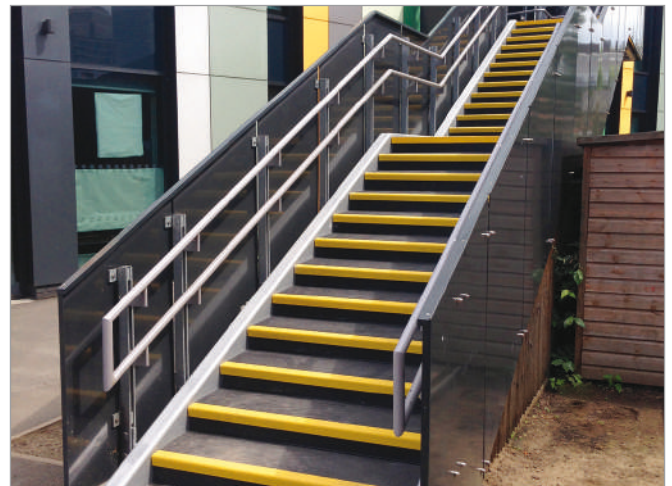
DDA compliant treads applied to stairs and landing areas.
