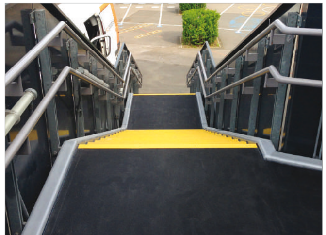
Stairs, ramps and walkways installation completed.
