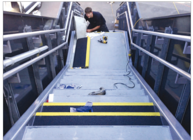
School stairway installation in progress.
